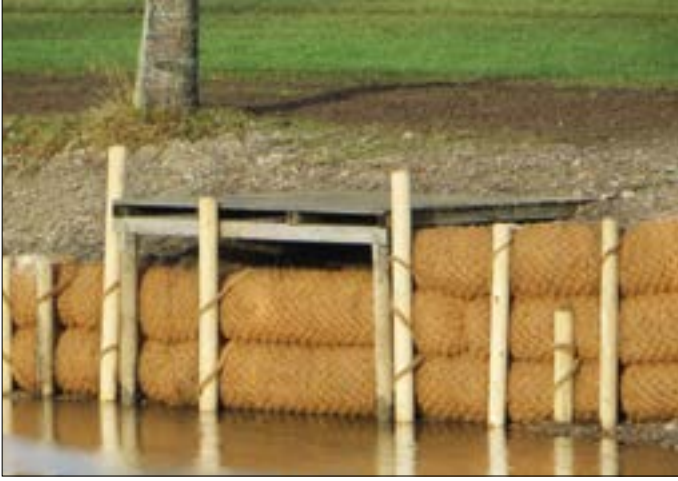
Figure 6: Georolls stacked at the edge of the bank with wooden stakes
