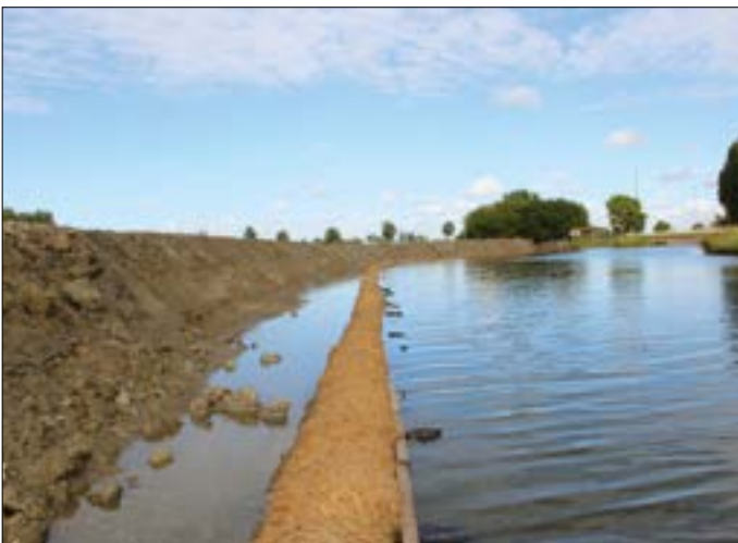
Figure 8: Georolls in a trench
