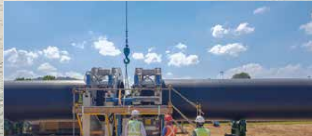
Site butt welding equipment for pipes and fittings up to OD 3500 mm.
