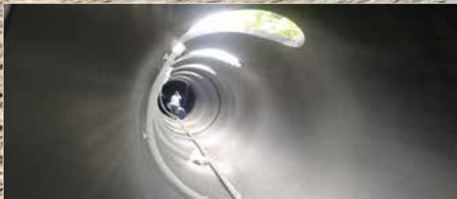
Project-specific chlorination systems to prevent bio-fouling of intake pipelines.
