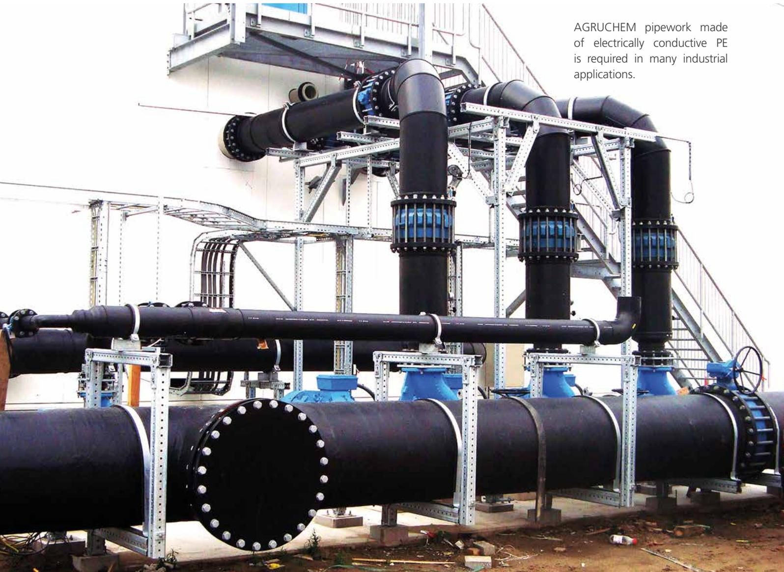
AGRUCHEM pipework made of electrically conductive PE is required in many industrial applications.
